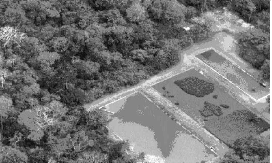
Figure 1 Biological sewage system at Robinson Club Baobab Source: Courtesy of TUI Hannover
